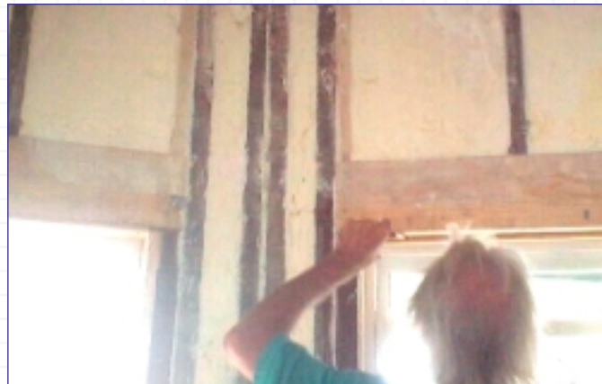
Icynene® is sprayed directly into the wall cavity. The foam softly expands to fill all of the cracks and crevices around the studs and window casings. Any excess foam is easily trimmed in preparation for drywall.
