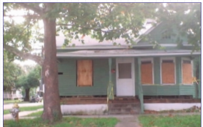
Icynene®, a high-performance insulation, was selected to address the homeowner's strong allergic sensitivity and reaction to mold and mildew.
