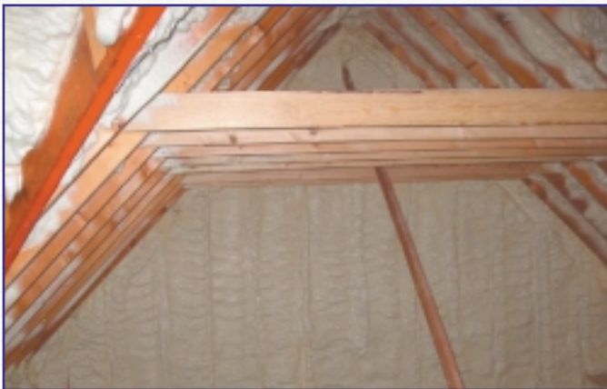
Areas that are considered difficult to insulate with conventional insulations are no obstacle for Icynene®. Cathedralized attics and gradient kitchen ceilings can be quickly and easily insulated.
